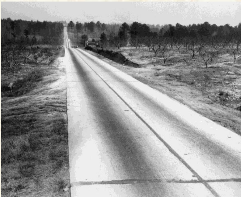
Concrete Dixie Highway in central Georgia, 1927.
